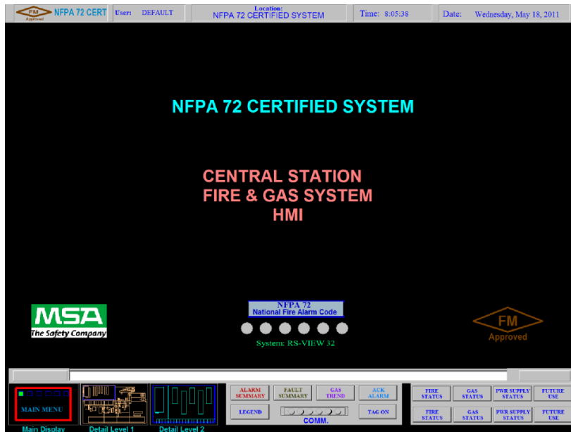
Figure 76: Central Station HMI Main Introduction Screen
